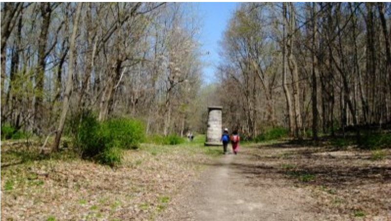
Ah, the 3rd ventilator we've passed on the OCA. The Croton Dam can't be far.
