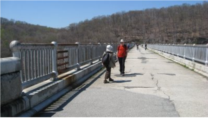
This bridge is the end of the trail. Wait 'til you see paydirt:
